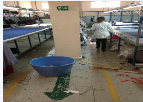
This evacuation route in the cutting section is obstructed by a beam.
