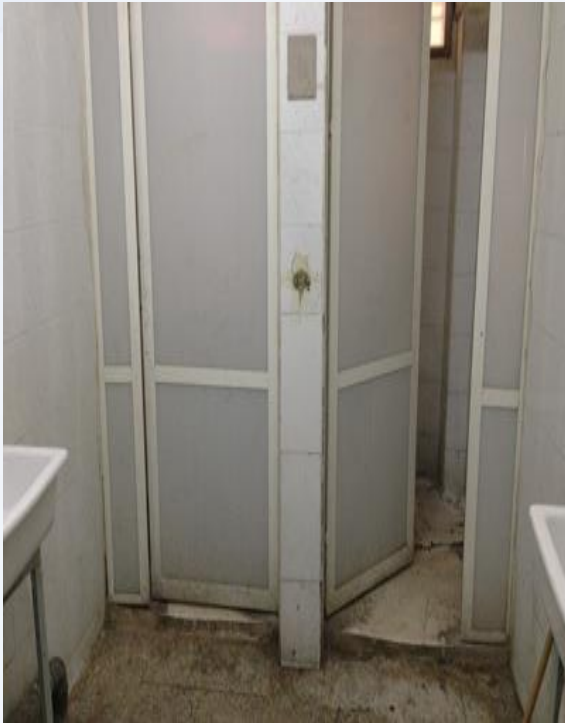
Toilets are sufficient in number and hygiene and permanently provided with water
